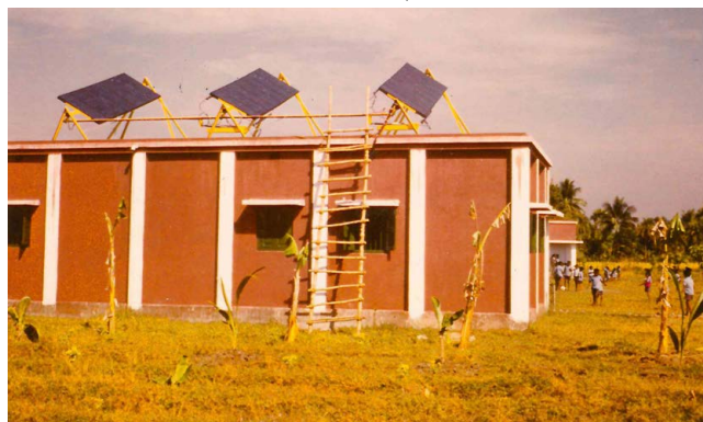
Solar installation of the Ananda School for irrigating the fields, 1987
